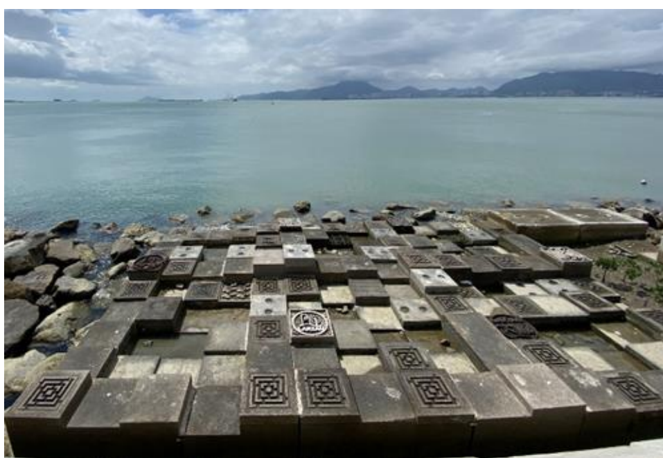
Example: Eco-shoreline at Tung Chung (bio-blocks)
