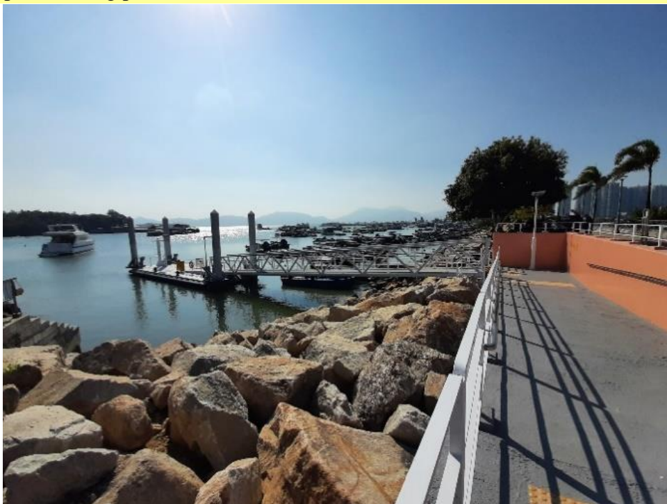
Example: Floating pontoon at Tuen Mun Area 27
